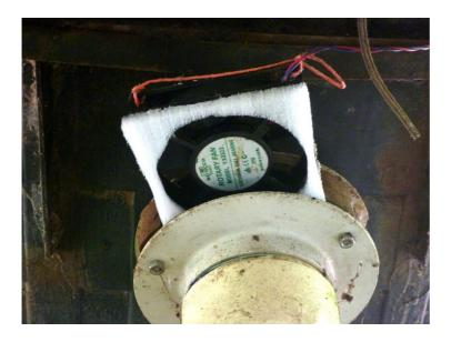
This fan is installed in a simple carrier, which allows easy removal. The white is a foam plastic gasket to reduce smells in the immediate vicinity of the fan (made out of packing foam and contact glued on).
